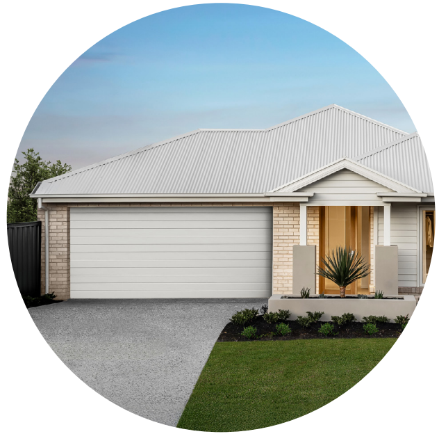
EXAMPLE OF GARAGE
